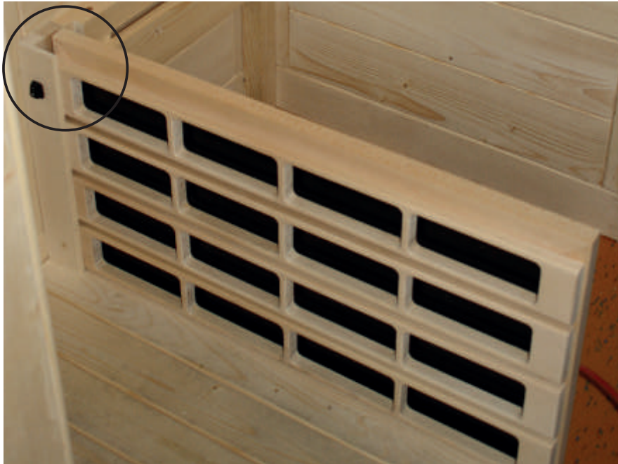
Fig. 34: Installation of the IR thermal plate VitaMy 164
