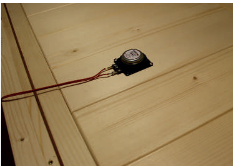
Fig. 47: Installation of the exciter
