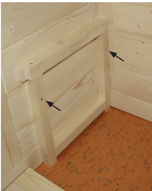
Fig. 32: Installation of the bench cushion
