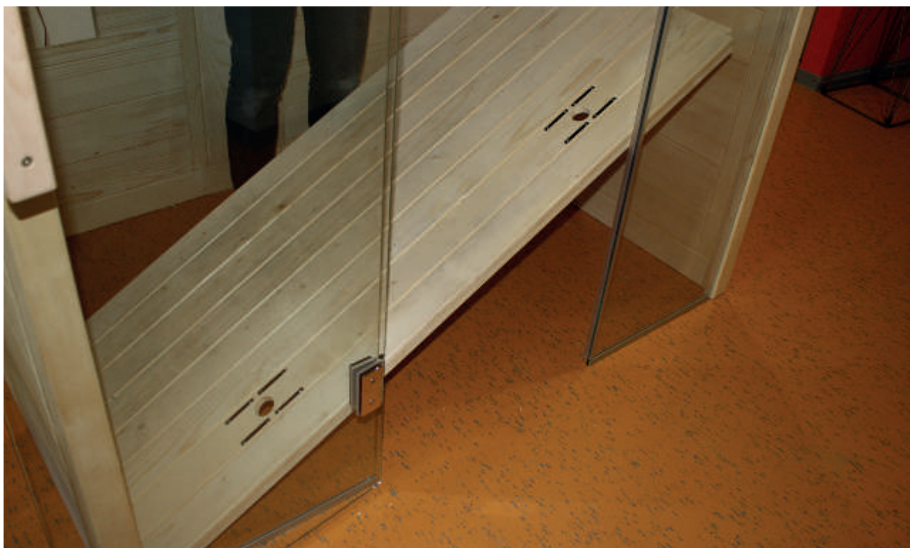
Fig. 28: Put the cabin floor in place
