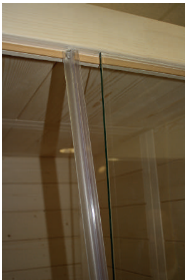
Fig. 20: Installing the door insulation strips
