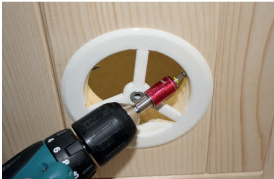
Fig. 36: Ventilation installation
