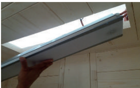
Fig. 50: Installing the colour light
