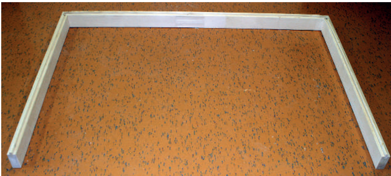
Fig. 1: Placing the three floor frame elements
