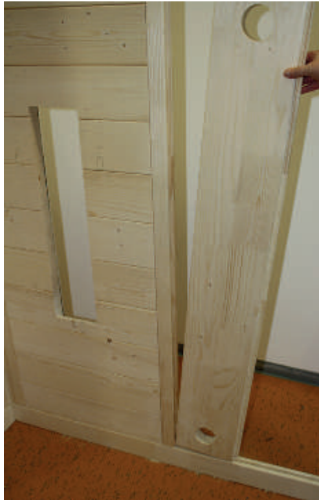
Fig. 6: Install the electrical element in place
