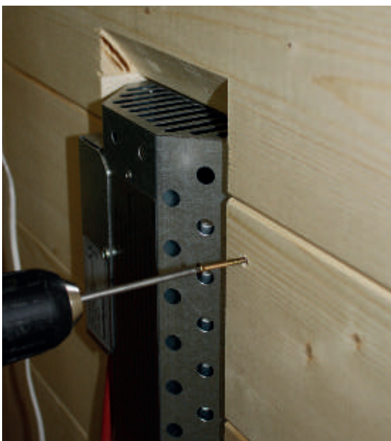
Fig. 42: Installing the read radiator blind
