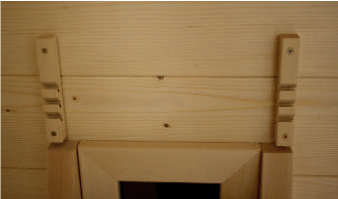
Fig. 54: Installation of the headrests
