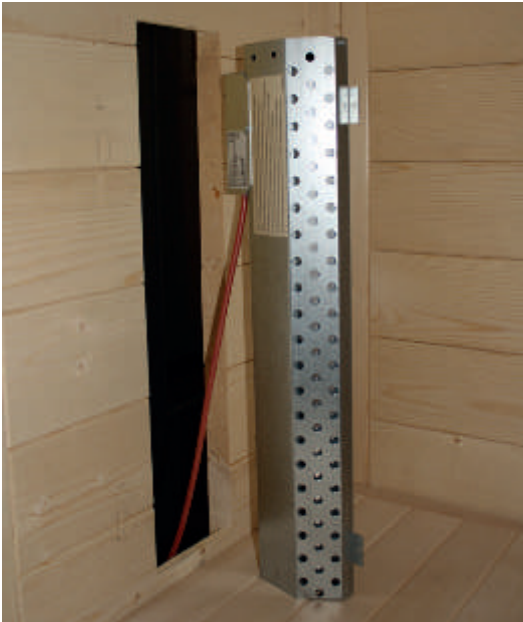
Fig. 41: Install the rear radiator (infrared radiator ECO 350)
