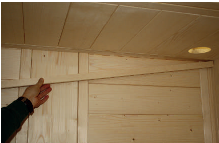
Fig. 37: Installation of the LED cover strip
