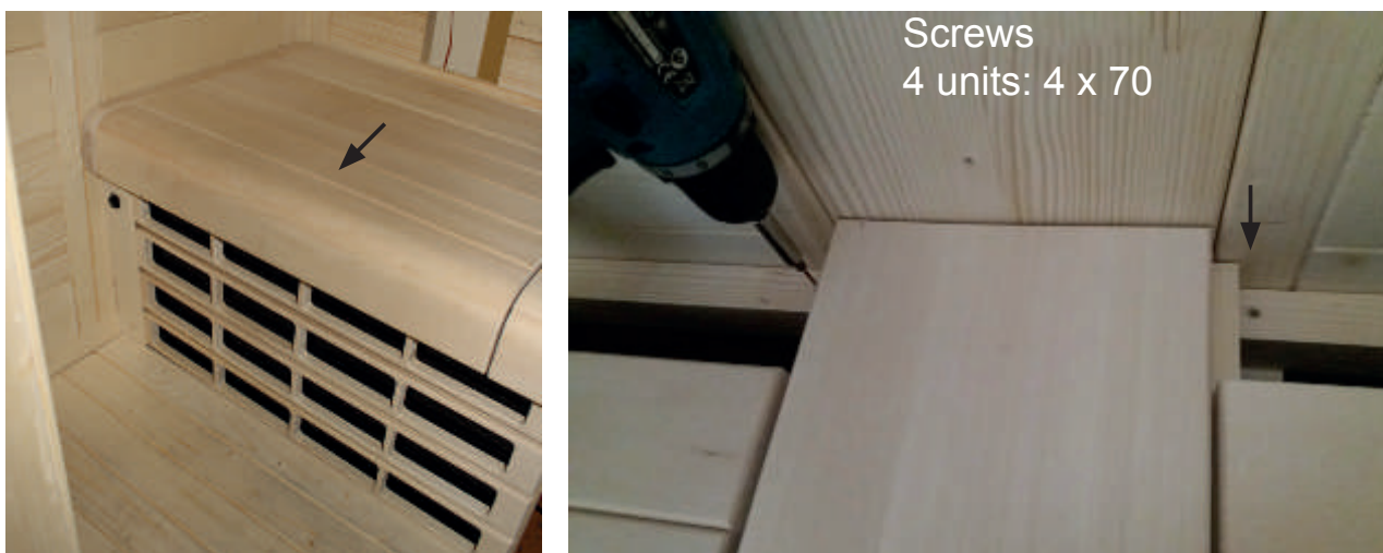
Fig. 51: Attaching the bench
