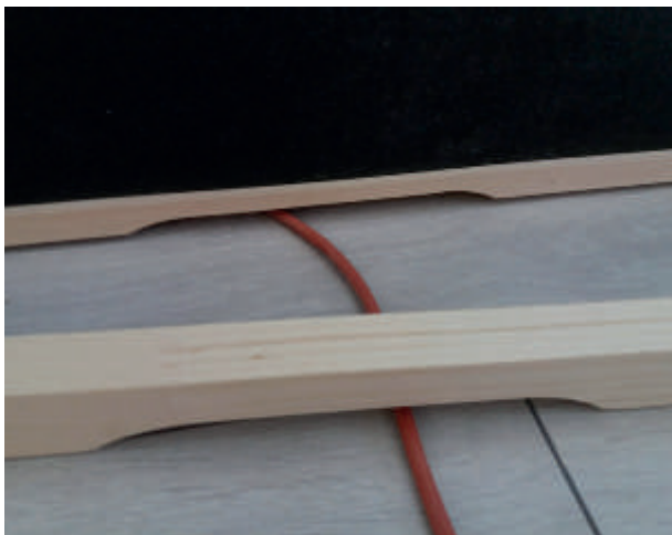
Fig. 35: Inserting the stiffener bar for the Vitamy IR thermal plates.
