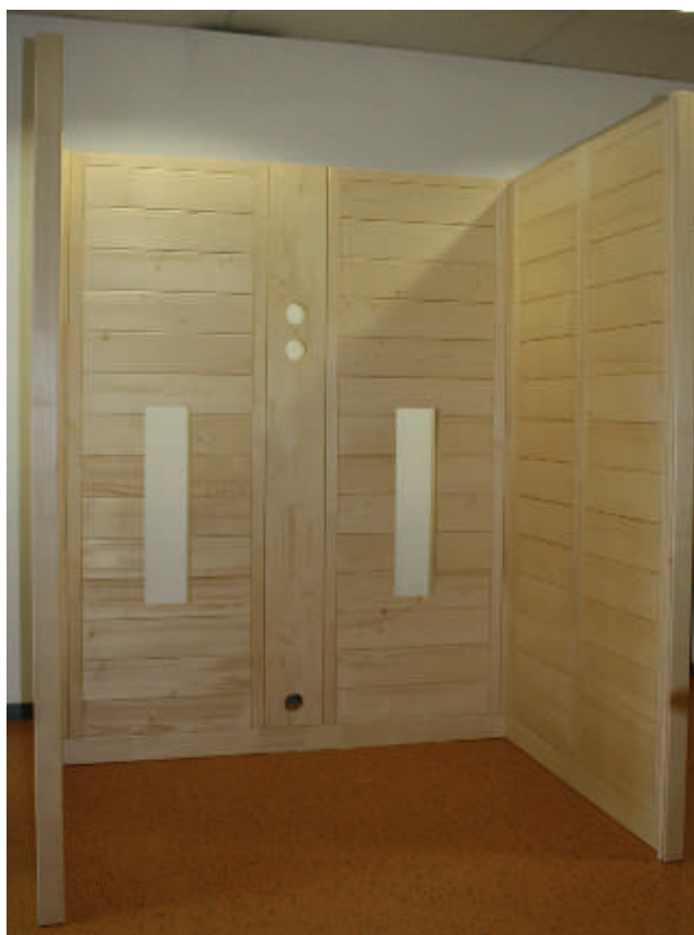
Fig. 10: Installed wall elements
