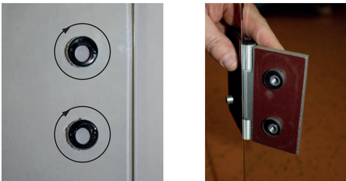
Fig. 22: Installation of Door Fitting 1
