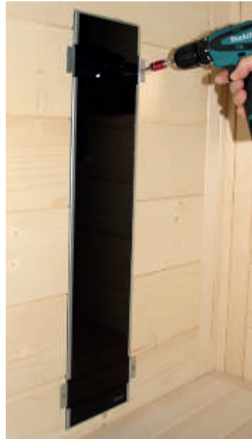
Fig. 41: Install the rear radiator (infrared radiator ECO 350)
