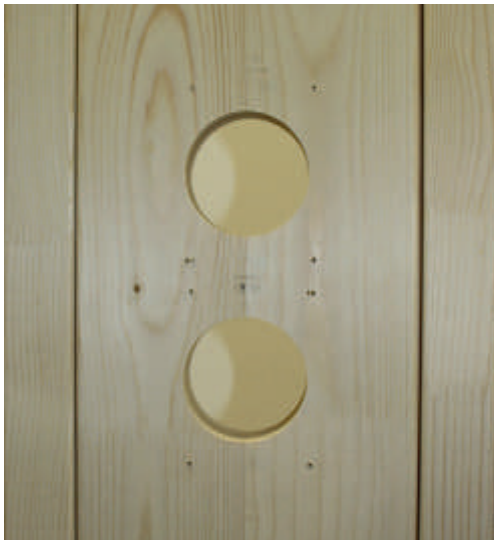
Fig. 46: Installing the control panel
