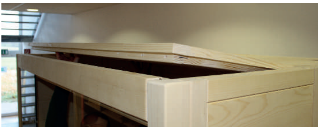
Fig. 18: Installing the roof element in the front
