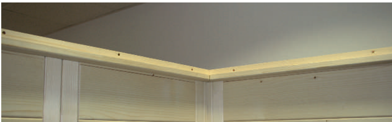
Fig. 16: Roof support slats
