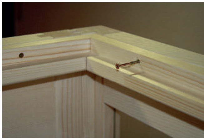
Fig. 14: Roof support slats installation
